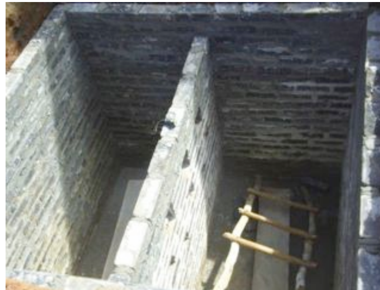
Transformation of plastic waste collected on the beach into construction bricks. Example of septic tank built with recycled waste bricks.
